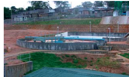
Project: Infrastructure development – Municipality, Knysna
