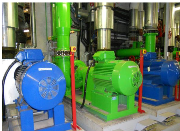
Chillers used for cooling the water
