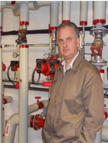
Noel getting an appreciation for the operation Climespace
